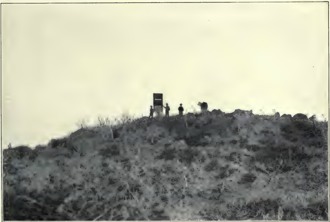
FIG. 6.—STATION BOSLEY SHOWING THE TYPE OF TARGET USED FOR THE SHORTER SECONDARY LINES.
